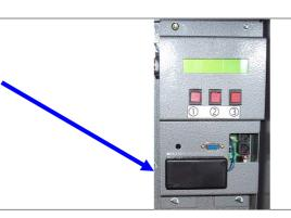
Feed the 24VAC wash start signal lines from your car wash through the hole in the Wash Open Interface Unit
