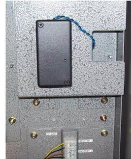
Feed the 24VAC wash start signal lines from your car wash through the hole in the Wash Open Interface Unit
